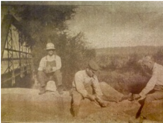
Part of Ed Cooney's work crew.
